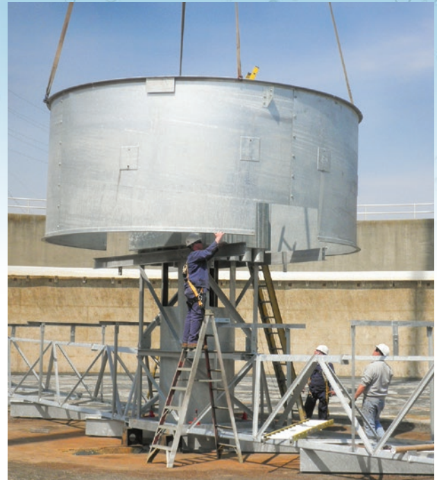
Rebuild of a Secondary Clarifier for municipal wastewater treatment
