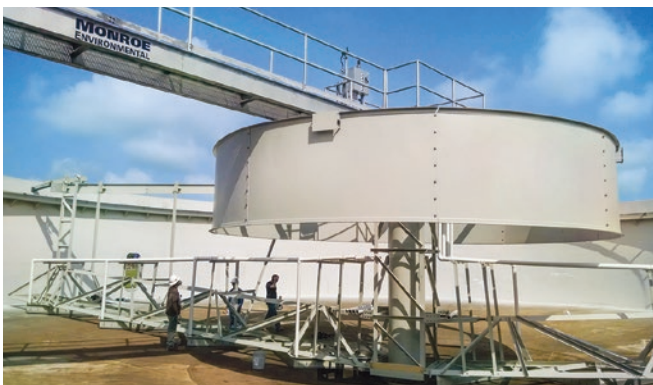
90 ft. diameter wastewater clarifier rebuild at chemical plant
