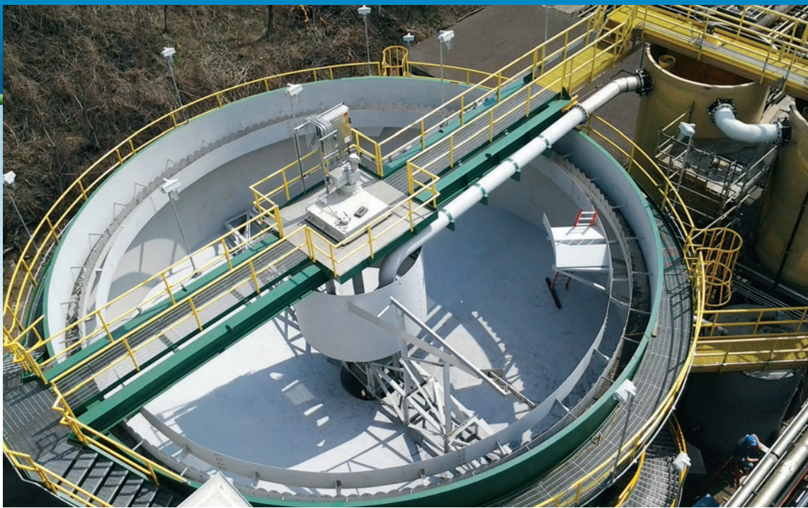
Above ground Circular Clarifier on legs with access bridge, walkway, and spiral staircase ready for startup at an industrial WWTP
