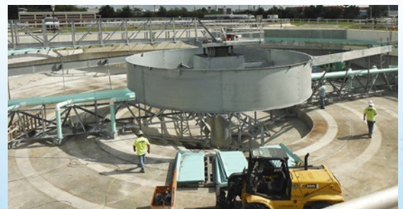
Installation of a 120 ft. Secondary Clarifier with riser pipes
