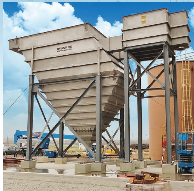
1,500 GPM stainless steel Vertical Clarifier with flash and flocculation tanks
