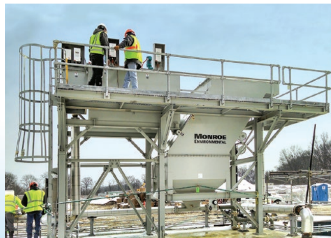
Installation of Vertical Clarifier for disc filter backwash with chemical mix tanks, access platform, ladder, and support structure
