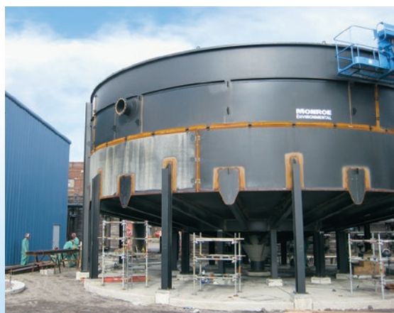
Field welding and final coating of an elevated steel tank clarifier
