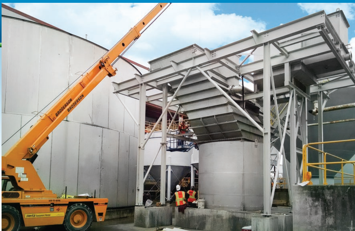
Vertical Plate Clarifier installation, stainless steel construction with integral thickening tank, support structure, and access platform
