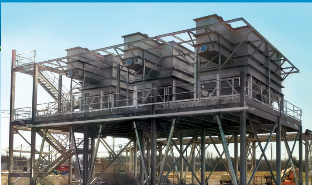
Three 1,000 GPM Horizontal Plate Clarifiers, stainless steel construction during installation at a plastics production plant
