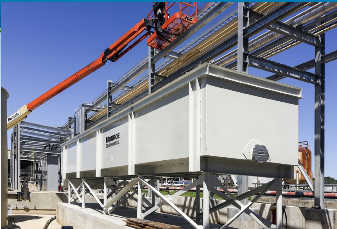
API Separator installation
