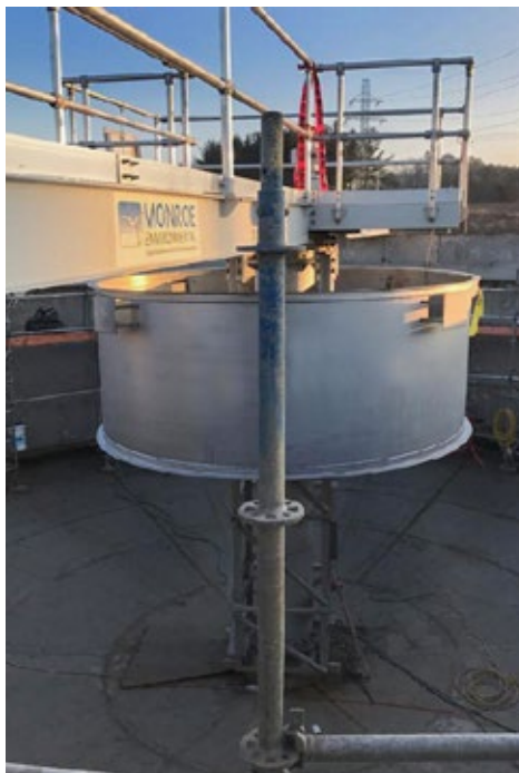
50 ft. diameter Circular Clarifier for leachate treatment at a superfund remediation site. The tank, mechanism, and internals were constructed from 316SS and the unit was designed to treat 1,600 GPM.
