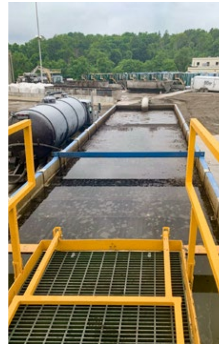
X-Flo Mobile Clarifier™ for treatment of hydraulic fracturing water (produced water, drilling mud, etc.) in the Marcellus Shale Formation. The 300 GPM system provided high capacity TSS and oil/water separation.
