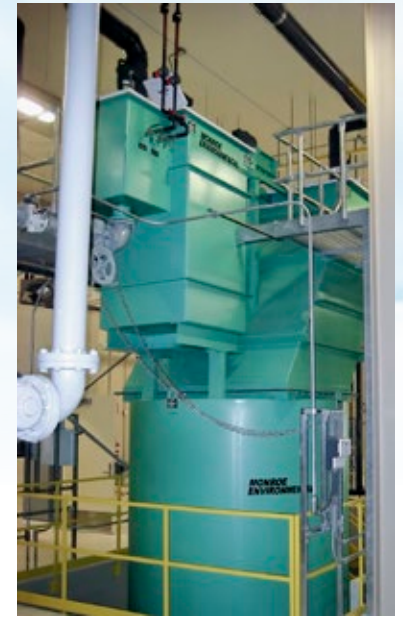
70 GPM Vertical Clarifier with flash and flocculation tanks, thickener, and FRP cover for landfill leachate treatment.
