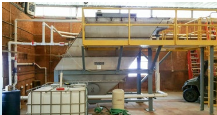
140 GPM Vertical Clarifier to treat leachate at a retired landfill. Monroe custom-designed a low-profile clarifier to meet the limited height requirement of the existing building.
