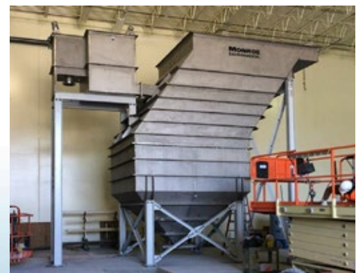
Vertical Plate Clarifier for leachate treatment at a landfill. The tank and plates were constructed from 316SS and the system was designed to treat 210 GPM.
