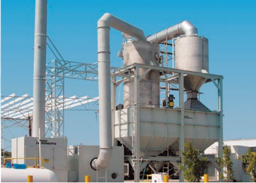
20,000 ACFM Multi-Stage Scrubbing System for waste incineration at 2,000°F including: ceramic-lined ductwork, Quench Tower, Venturi Scrubber, Packed Tower Scrubber, carbon filter, fan, and discharge stack. Regulations met included SO 2 , HCl, PM, mercury, metals, PCDD/PCDF, etc.
