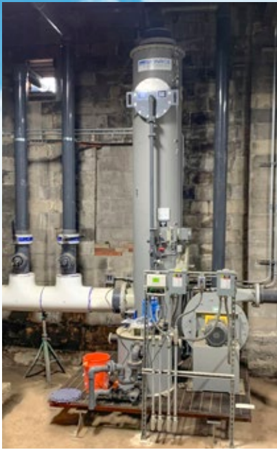
Packed Tower Scrubber to absorb H 2 S fumes and other odors from an industrial waste treatment process. The Scrubber exhausts the storage tanks and a Monroe Vertical Plate Clarifier that is part of the site's PFAS treatment system.
