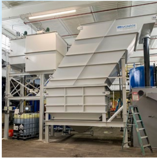
Vertical Plate Clarifier to remove heavy metals and TSS in PFAS treatment process. The 500 GPM Clarifier is equipped with a pyramid sludge hopper, flash mix and flocculation tanks, and chemical mixers.
