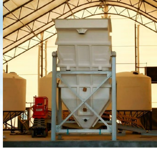
Vertical Plate Clarifier to remove mercury and humic acid from incoming groundwater. FRP construction was selected to withstand corrosion from the highly acidic water, and a conservative hydraulic loading rate was selected to allow for proper settling of the tricky solids.
