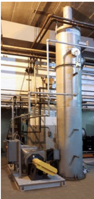
Air Stripper to remove ammonia from ethylene glycol for an industrial solvents facility. To increase the purity of recycled ethylene glycol, it was heated to 150°F prior to the stripper. This is favorable for ammonia stripping due to its increased vapor pressure at the higher temperature.
