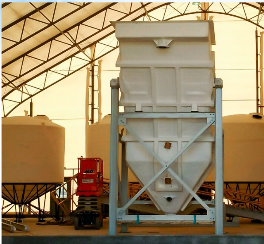
UV-resistant polypropylene modular laminar plate cartridges were recommended to help increase flow rate from 950 GPM to 1,350 GPM
