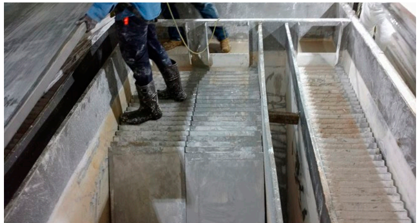
After: Lamella plates installed after new supports for internal structural and process deficiencies were addressed.
