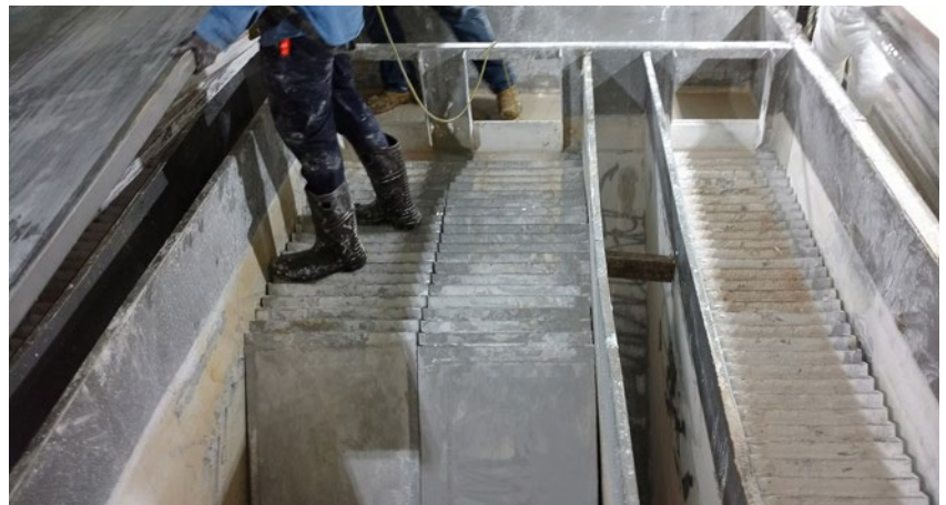
After: Lamella plates installed after new supports for internal structural and process deficiencies were addressed.
