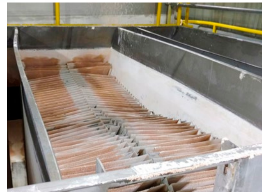
Before: Lamella plate clarifier with internal components that were warped, buckling, and in danger of collapsing.
