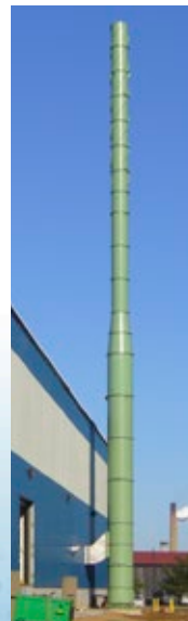
35,000 ACFM Multi-Stage Mist Collection system for production expansion at stainless steel finishing plant. The system included a high-efficiency collector, ID fan, ductwork, controls, and a 145 ft. free standing stack.
