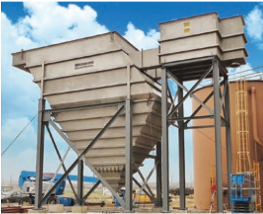
Lamella Plate Vertical Clarifier to remove iron and nickel hydroxides from metal finishing wastewater. The 1,533 GPM unit was constructed of 304SS, equipped with flash mixing and flocculation tanks, and provided over 3,900 ft 2 of settling area.
