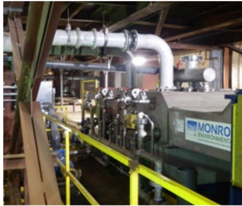
Wastewater treatment and steel coil line upgrade for a galvanizing plant. Monroe provided engineering, integration, and oversight for the redesign, retrofit, and installation of the multi-million dollar upgrade. New equipment included insulated and heated oil separation and recovery tanks, steel coil quench tank, liquid filters, system sumps, purge tanks, transfer pumps, piping, valves, controls, and a new fume exhaust system.
