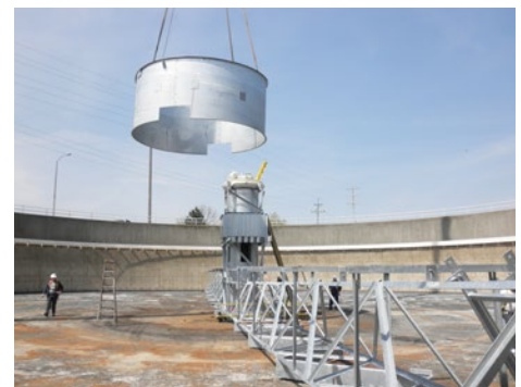
Installation of rebuild components
