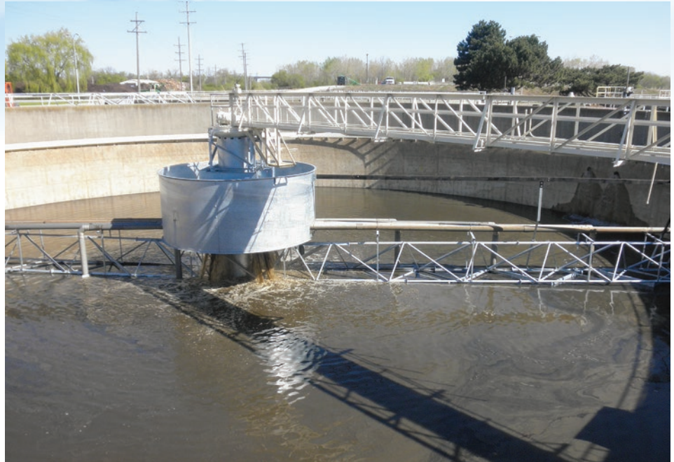
The rebuilt Secondary Clarifier back in service.
