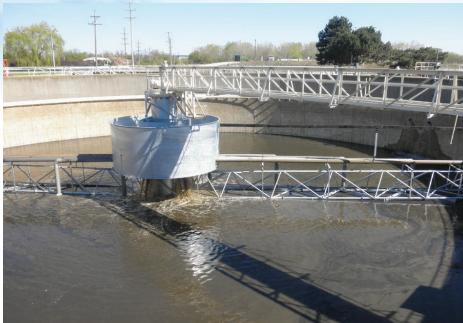
The rebuilt Secondary Clarifier back in service.
