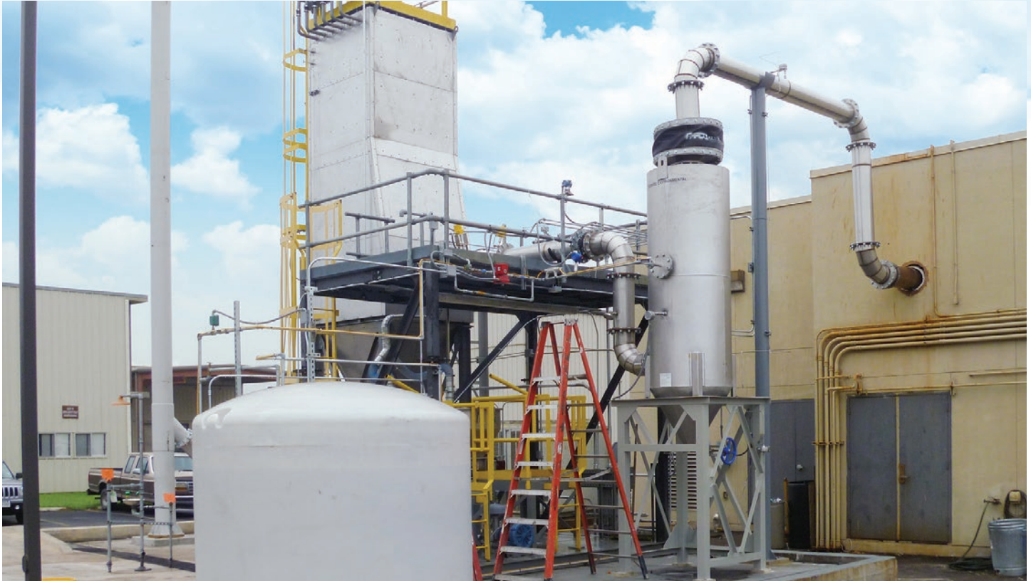
Quench Tower for gas conditioning prior to baghouse dust collector, AL6XN alloy construction
