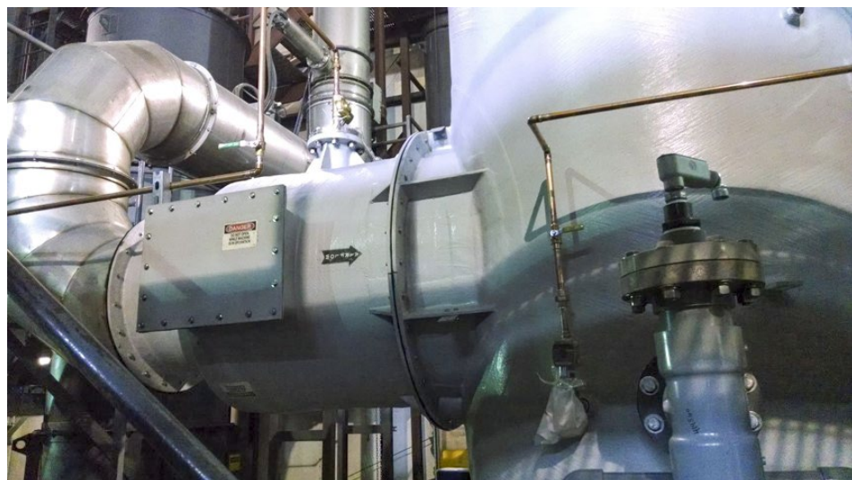
Inlet duct quench with horizontal spray configuration
