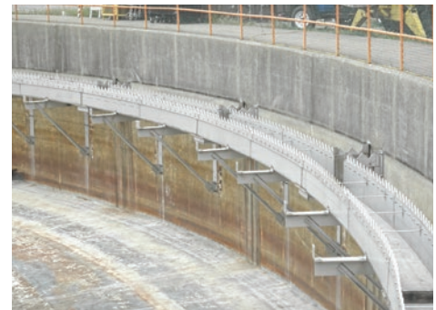
Clarifier with stainless steel weirs after rebuild
