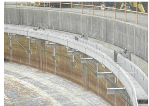
Clarifier with stainless steel weirs after rebuild
