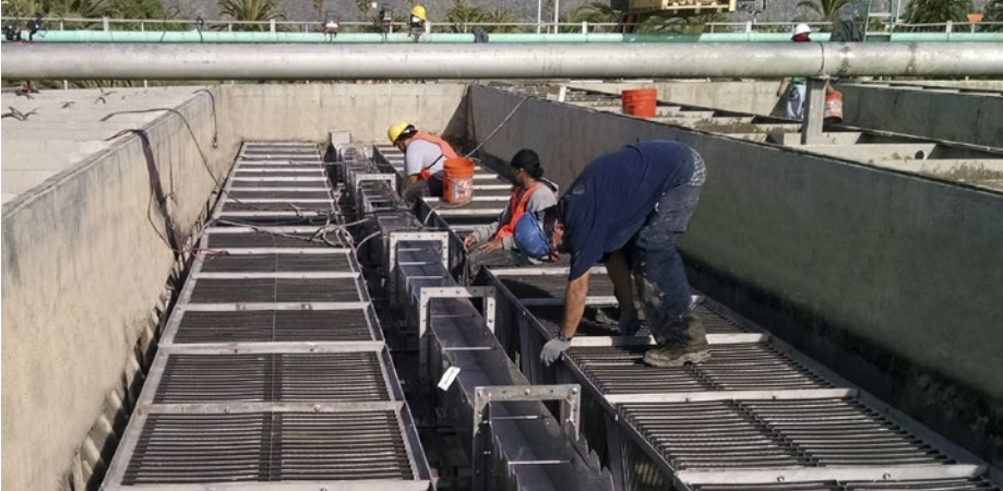
Plate Settlers and collection launders during installation.
