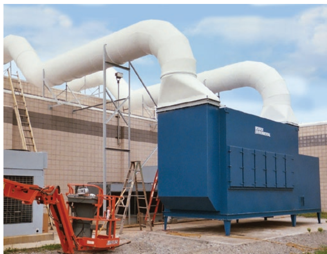
Custom designed ductwork system with supports for recirculating climate controlled clean air after filtration through a 30,000 CFM Mist Collector
