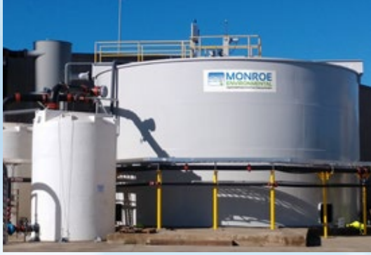
40 ft. diameter Circular Clarifier for wastewater treatment at a specialty minerals plant. Clarifier was elevated on legs with a tank skirt that went to grade for additional support. Monroe provided the complete clarifier system including tank, drive, mechanism, bridge, and access platform with installation on a turnkey basis. The unit was rated for 1,000 GPM.
