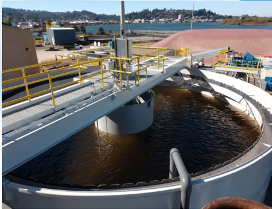
40 ft. diameter Circular Clarifier for wastewater treatment at a specialty minerals plant. Clarifier was elevated on legs with a tank skirt that went to grade for additional support. Monroe provided the complete clarifier system including tank, drive, mechanism, bridge, and access platform with installation on a turnkey basis. The unit was rated for 1,000 GPM.
