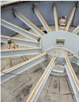
40 ft. diameter Circular Clarifier for wastewater treatment at a specialty minerals plant. Clarifier was elevated on legs with a tank skirt that went to grade for additional support. Monroe provided the complete clarifier system including tank, drive, mechanism, bridge, and access platform with installation on a turnkey basis. The unit was rated for 1,000 GPM.
