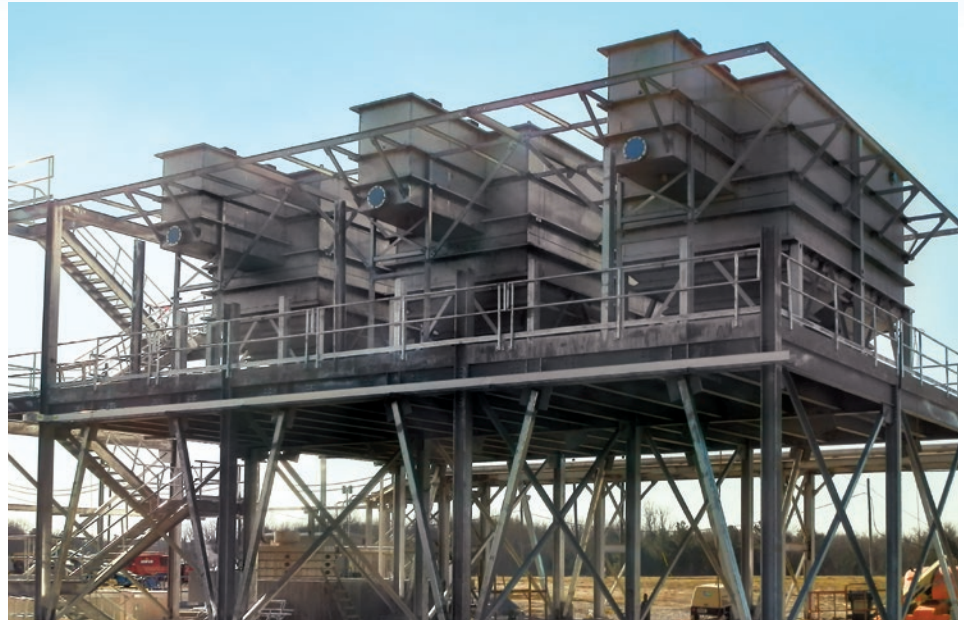
Three 1,000 GPM Horizontal Plate Clarifiers, stainless steel construction during installation at a plastics production plant
