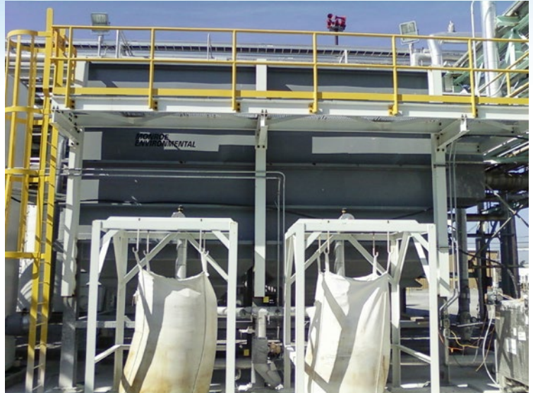
600 GPM Horizontal Clarifier with dual pyramid hoppers
