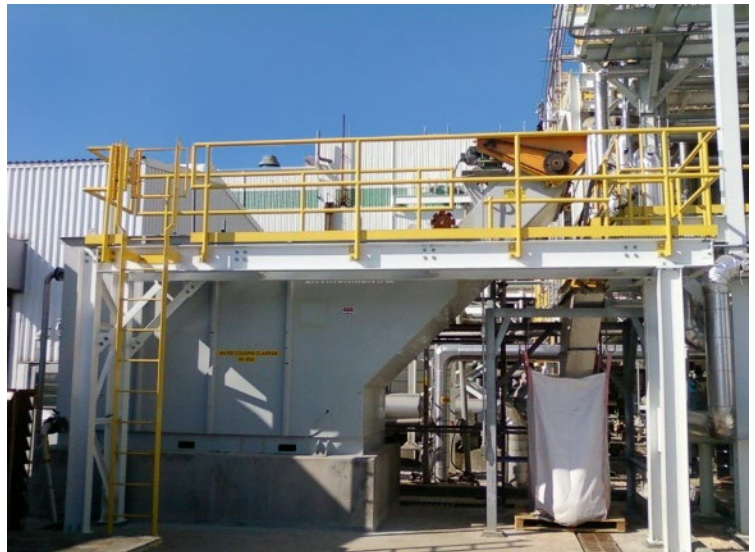
150 GPM Horizontal Clarifier with drag conveyor
