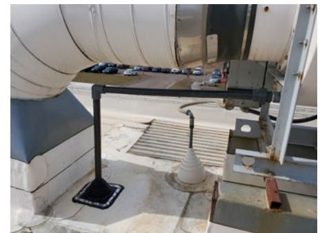
Drain lines from the fan were installed, allowing a path for acid to drain back into the scrubber.
