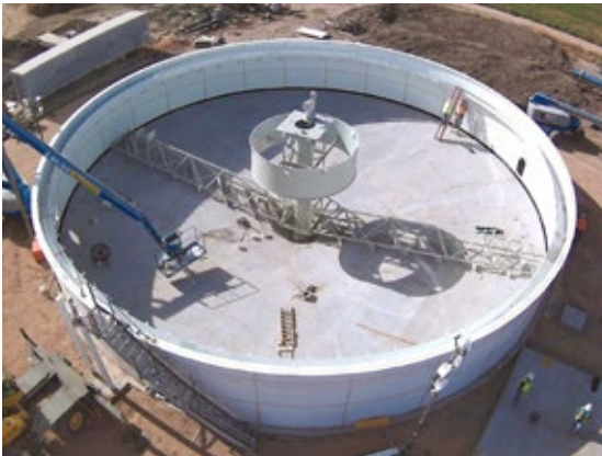
85 ft. diameter Circular Clarifier to process wastewater at a dairy farm. The Monroe supplied mechanism was installed in a bolted steel tank with concrete floor. Clarifier was rated for up to 2,000 GPM.
