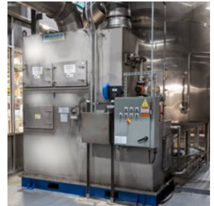
Dual Throat Venturi Scrubber to handle sticky, water soluble particulate for a beverage producer. The system was rated for 6,600 CFM and met the 99%+ removal efficiency of particles greater than 10 micron.
