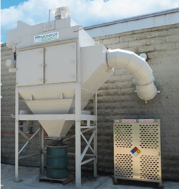
6,000 CFM Cartridge Dust Collector with inlet duct and storage drum exhausting a sandblasting and paint spraying operation
