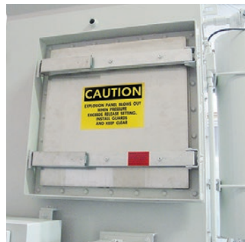
Dust Collector explosion panel
