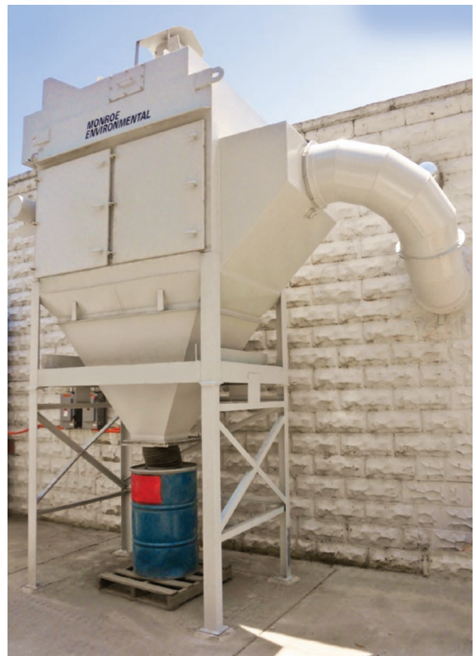
Dust Collector for sandblasting and painting operation
