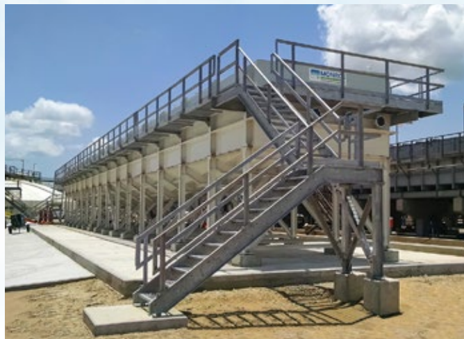
A custom Monroe API Oil Water Separator provides primary oil, water, and solids separation prior to downstream biological treatment for a gulf coast refinery. The unit was 150 ft. long and included a cover, explosion protection vents, and was built to API 421 standards.
