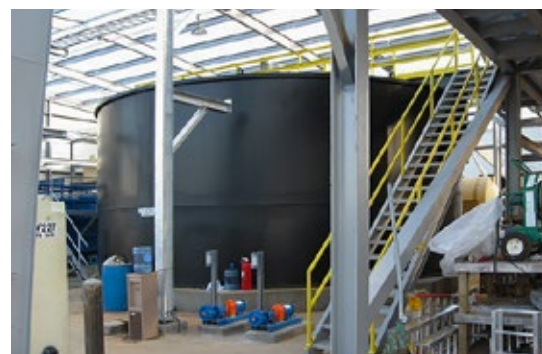
30 ft. diameter Circular Clarifier to treat wastewater at a fluoropolymer plant. Monroe provided the complete clarifier system, including tank, drive, mechanism, bridge, and access platform with installation on a turnkey basis.
