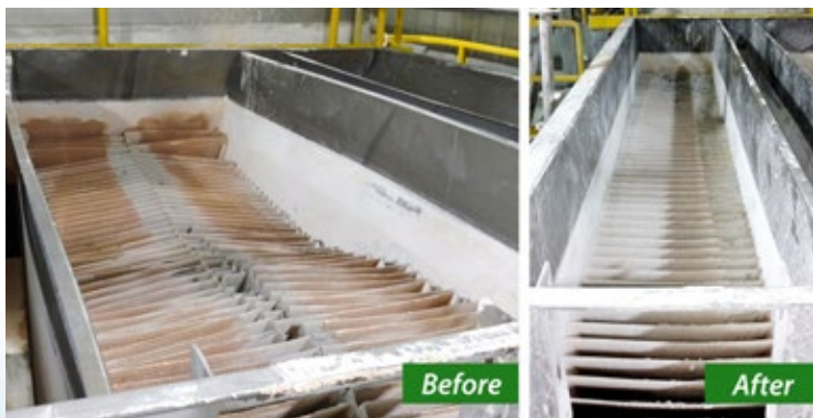
Retrofit of two Lamella-type Plate Clarifiers at a chemical plant. A competitor's clarifier was insufficiently designed to handle process temperatures and was warping and buckling, causing safety and process hazards. Monroe gutted the clarifier and installed new supports and plates to allow the unit to operate properly, saving the plant over $200,000 versus replacing the clarifier.
