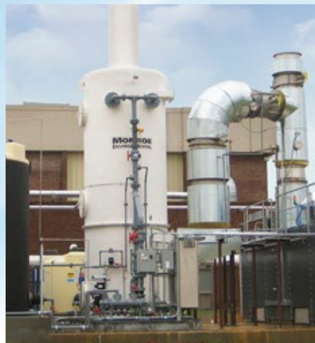
Wet Scrubber treats HCl & Cl 2 exhaust from RTO: A Monroe Wet Scrubber system was selected to capture and neutralize the toxic gases at a pharmaceutical manufacturing plant.
