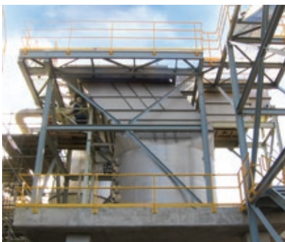
Lamella Plate Vertical Clarifier for the reduction of cobalt hydroxides from a process water stream at a petrochemical plant.
