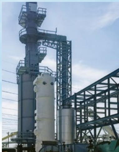
Quench Tower and SO 2 Scrubber for boiler expansion: A chemical plant that produces coal tar pitch was expanding operations and needed to control flue gas emissions from a new boiler.
