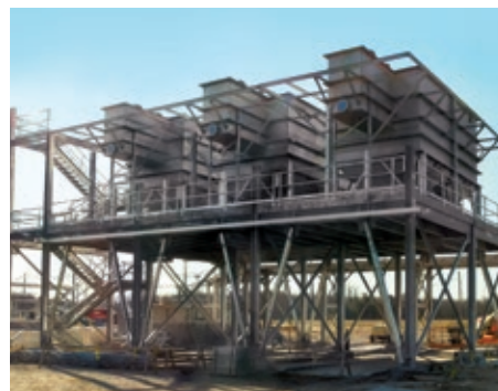
Horizontal Plate Clarifiers provide water re-use for resins plant: Separates PVC resins and other solids from large volumes of process water to allow for re-use.
