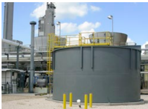
Solids Contact Clarifier for midstream oil and gas facility to process river water – softening and lowering total suspended solids, metals, and turbidity – for use in the plant.
