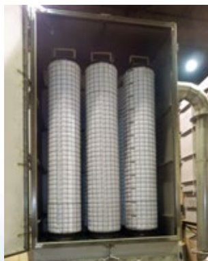
Fiber Bed Mist Collectors for asphalt storage terminal to control PM 2.5 particulate, fumes, mist, and vapors exhausted from its heated asphalt storage tanks. Downstream H 2 S adsorption vessels would plug and fail if these pollutants were not removed. The mist and vapors were very fine, requiring filtration equipment capable of removing submicron particulate.
