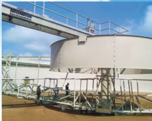
Secondary Clarifier for polymer plant: Rebuilt and upgraded to maximize sludge removal for 90 ft. diameter Circular Clarifier capable of processing over 2 million gallons per day.
