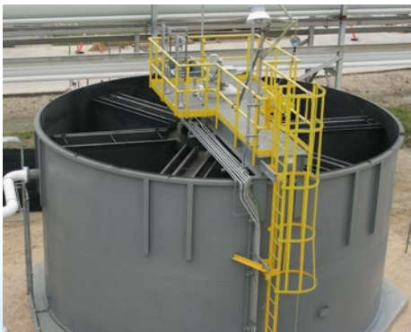
High rate Solids Contact Clarifier
