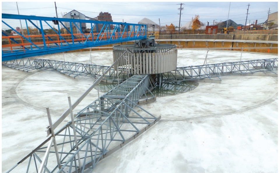
Above: 250 ft. diameter spiral scraper type Circular Clarifier at a municipal WWTP
