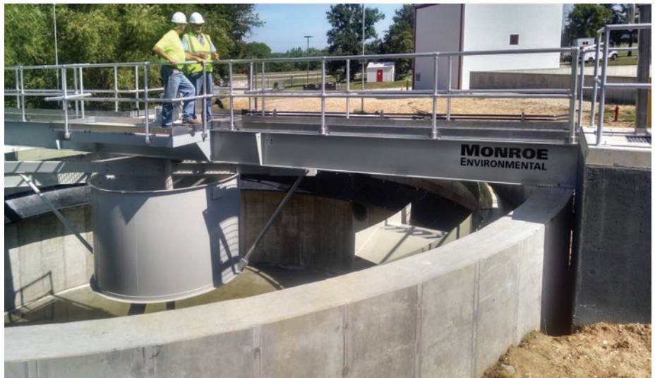
In ground Circular Clarifier at a beverage manufacturing plant prior to start up
