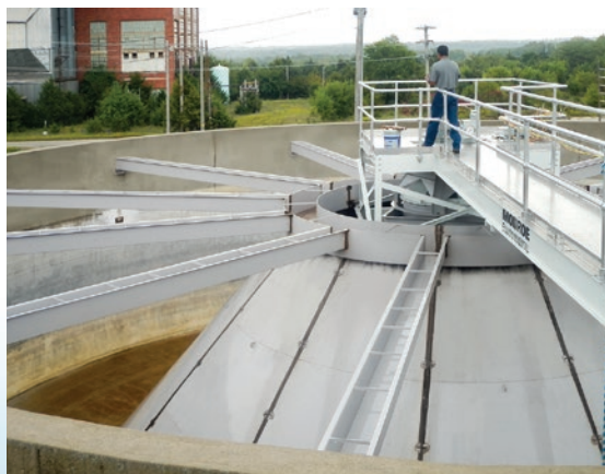
Above: 250 ft. diameter spiral scraper type Circular Clarifier at a municipal WWTP
