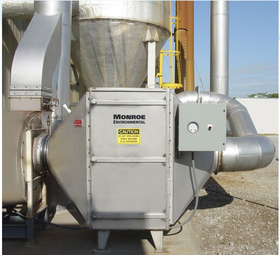
8,000 CFM Carbon Tray Adsorber for a recycling facility, shop assembled with stainless steel housing and differential pressure gauge
