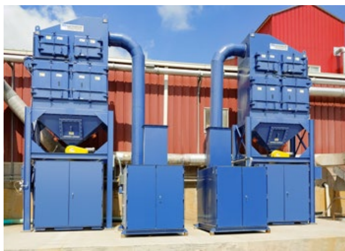
High efficiency Cartridge Dust Collectors for brick and terra cotta manufacturing facility to exhaust mills and protect employees from exposure to crystalline silica dust. The plant had several material transfer and processing stations, each requiring a custom hood, ductwork, collector, and control system.
