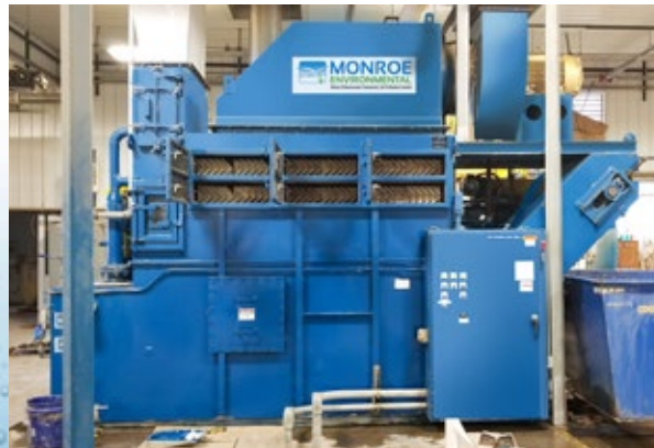
28,000 ACFM Venturi Scrubber , 304SS construction, for PM removal from FRP panel manufacturing process. The system included venturi throat, integral sump and separator, chevron mist eliminator, recirculation pumps, solids drag conveyor, and controls.
