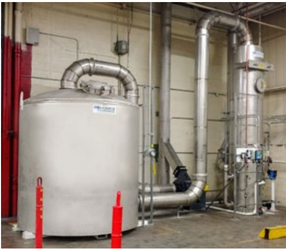
Multi-Stage Scrubbing System to remove H 2 S and VOCs from rubber vulcanizing process exhaust. System included Packed Tower Scrubber, Carbon Adsorber, ID fan, stack and ductwork, all 304SS construction and was rated for 3,000 ACFM.
