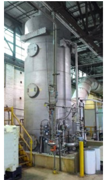
Wet Scrubber treats nitric acid from dryer at ceramics plant. The 26,400 ACFM system can simultaneously cool the incoming gas temperature, control the acid fumes, and withstand the corrosive environment as it captures and neutralizes hot, nitric acid emissions from a production dryer.
