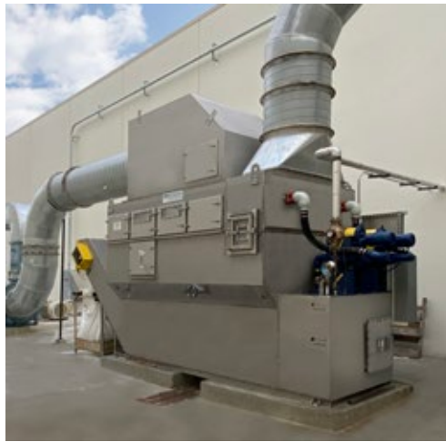
28,000 ACFM Venturi Scrubber , 304SS construction, for PM removal from FRP panel manufacturing process. The system included venturi throat, integral sump and separator, chevron mist eliminator, recirculation pumps, solids drag conveyor, and controls.
