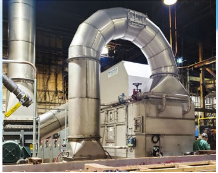
40,000 ACFM Dual Throat Venturi Scrubber for collection of PM from insulation drying ovens. Unit was constructed of 304SS and included venturi scrubber with recirculation pump, integral liquid reservoir, chevron demister, drag conveyor for solids removal, fan, piping, valves, instruments, and controls.
