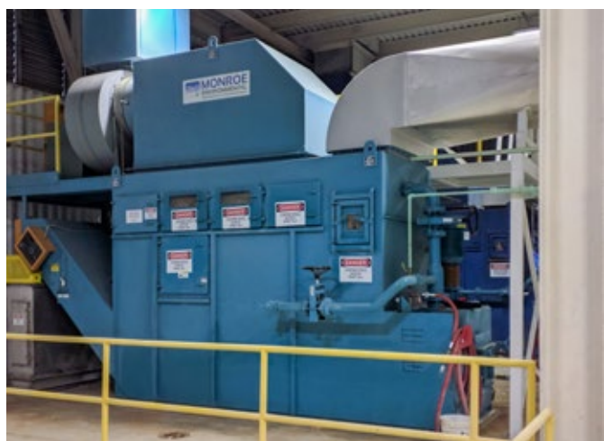
Dual Throat Venturi Scrubber to exhaust dryer for insulation and panel board manufacturing. The 18,000 ACFM unit with drag conveyor captures fumes and PM.
