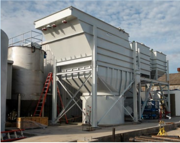
Vertical Plate Clarifier with three pretreatment mixing tanks to clarify process water at specialty insulation manufacturing plant. The system included an integral sludge thickener and was rated for 750 GPM.
