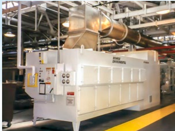
Spiral Tube Mist Collector exhausting multiple machining booths at an automotive engine manufacturing plant. Central systems exhausting multiple booths have lower life-cycle costs versus individual collectors.
