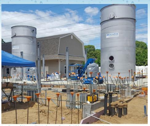
Installation of (2)1,400 GPM Air Stripping Towers for VOC treatment upgrades.
