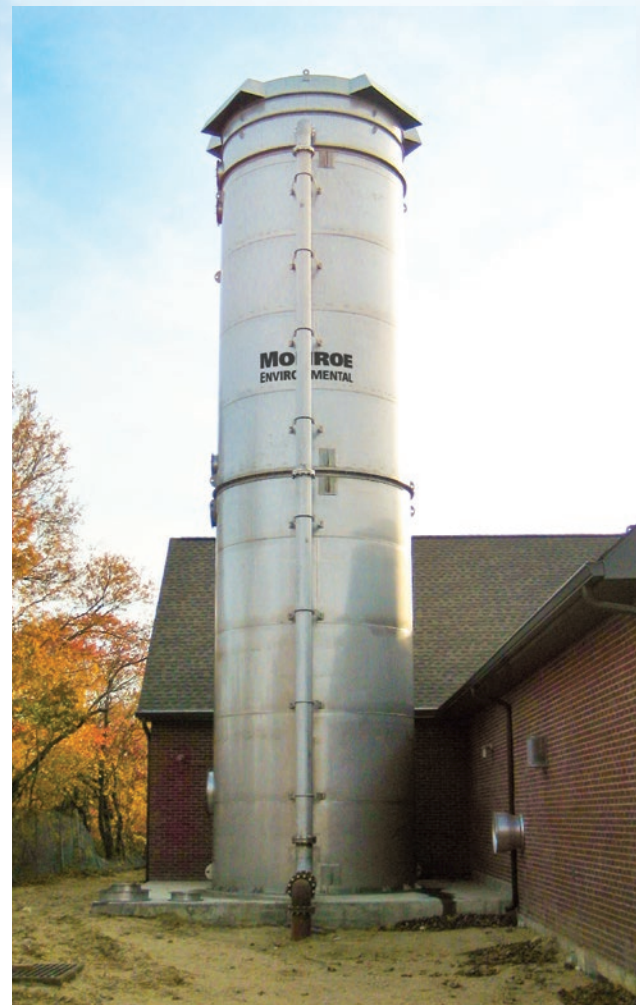
Air Stripper for VOC removal – Monroe's engineered unique air discharge arrangement reduces the noise allowing for quieter operation.
