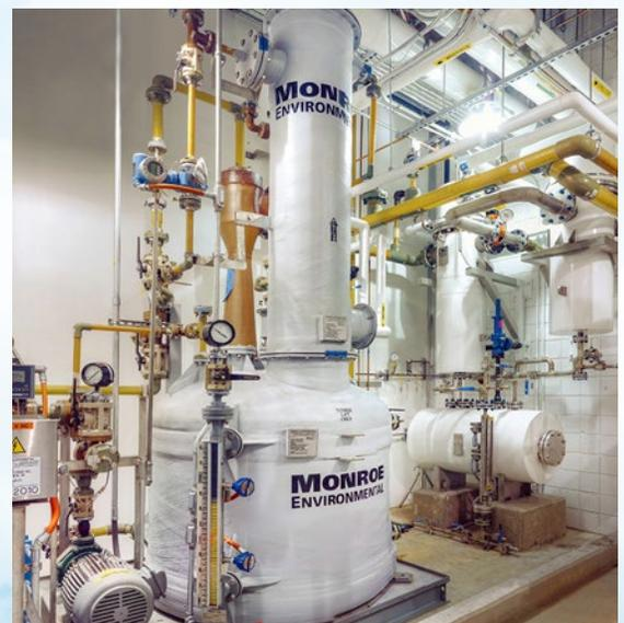
*Two-stage wet scrubbing system with eductor venturi and packed tower for HCl and SO<sub>2</sub> reduction from pharmaceutical manufacturing process exhaust*
