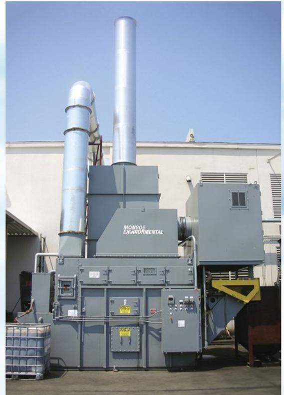
15,000 CFM Scrubbing System to condense and reclaim vaporized grease and remove hydrocarbon fumes from a chemical manufacturing process. The system includes a Dual Throat Venturi Scrubber with drag conveyor, Oil Recovery Unit, and Packed Bed Scrubber for odor control.
