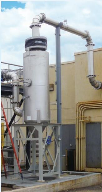
*Quench Tower for gas conditioning prior to baghouse dust collector, AL6XN alloy construction*
