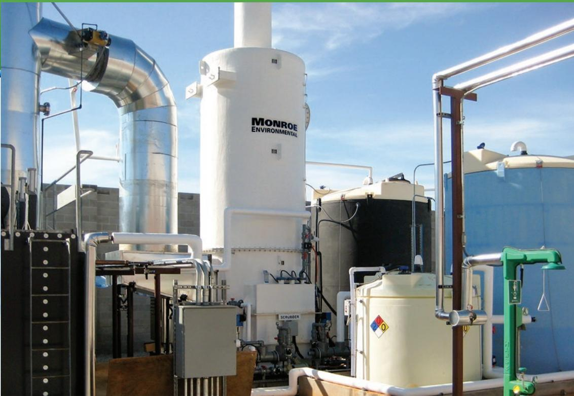
12,500 CFM scrubbing system for HCl and Cl<sub>2</sub> removal from RTO exhaust
