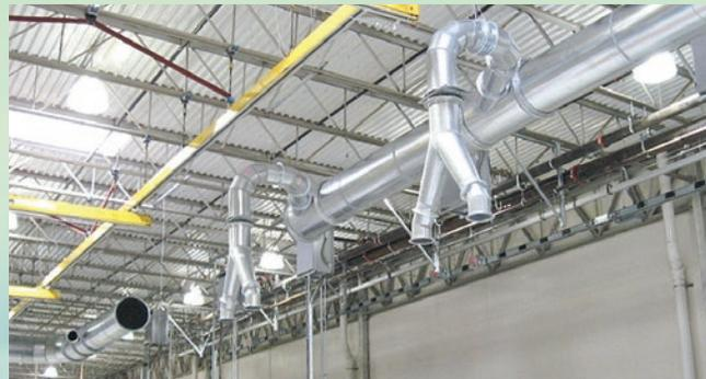
Tapered ductwork system with individual source hoods for multiple Oil Mist Collectors on a high production machining line
