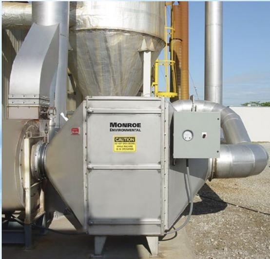
Tray-type Carbon Adsorber for odor control at a grainery
