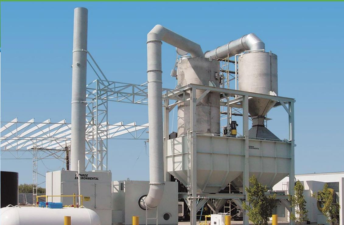
20,000 CFM Multi-Stage Scrubbing System for solid waste incineration process. (From right): Ceramic-lined inlet duct, rapid water quench, adjustable Venturi Scrubber, liquid clarification tanks, Packed Bed Scrubber, and Carbon Adsorber.
