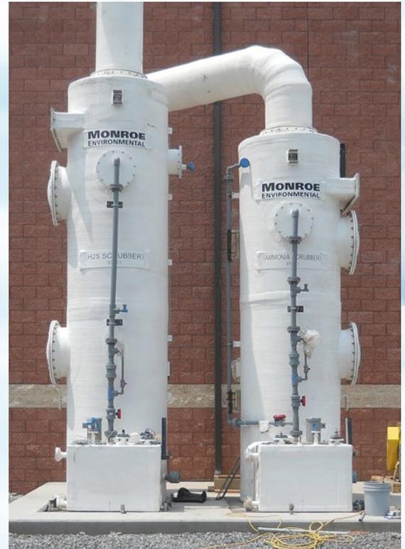
*Two-stage Packed Bed Scrubber to remove acids and alkalines from dryer exhaust gas*
