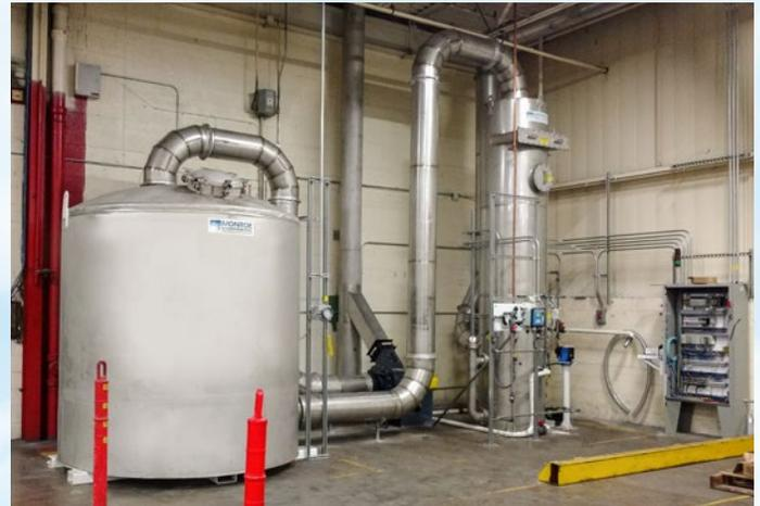
Packed Tower Scrubber followed by Carbon Adsorber for H<sub>2</sub>S and VOC reduction from a rubber manufacturing process
