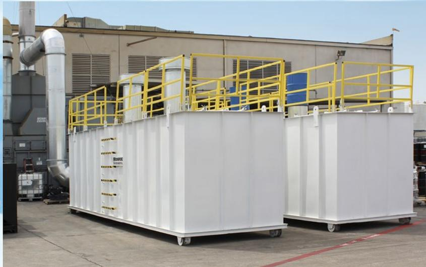
Two 15,000 CFM Deep Bed Carbon Adsorbers, mild steel construction with specialty exhaust stacks for odor control at a grease manufacturing facility
