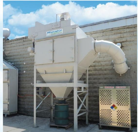
6,000 CFM Cartridge Dust Collector with inlet duct and storage drum exhausting a sandblasting and paint spraying operation
