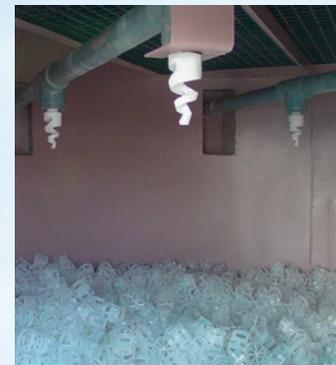
Non-plugging spray nozzles above bed of loose fill polypropylene packing
