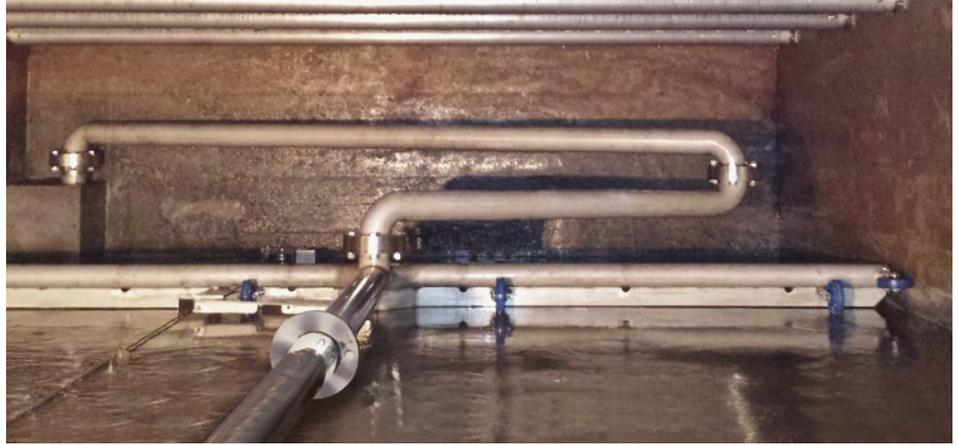
The Monroe Sludge Collector is the perfect compliment to the highly efficient Monroe Plate Settlers for potable water treatment. The unit can also be provided separately should your plant only require a more efficient settled solids removal system.
